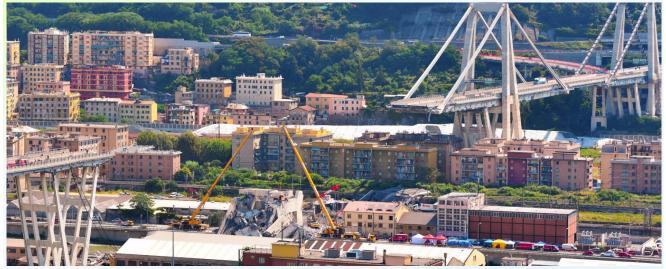
On 14 August 2018, during a rainstorm, a span of the 1182 m long and 45 m heigh Morandi bridge in Genoa broke. The bridge collapse caused 43 death.
